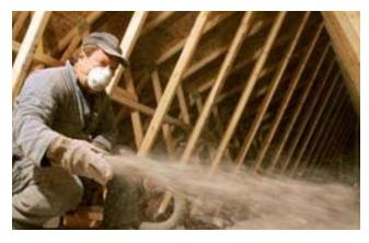
Installation costs vary. Loose-fill cellulose insulation is less expensive to install than batt insulation though. When installed properly, loose-fill cellulose insulation also provides better coverage.
